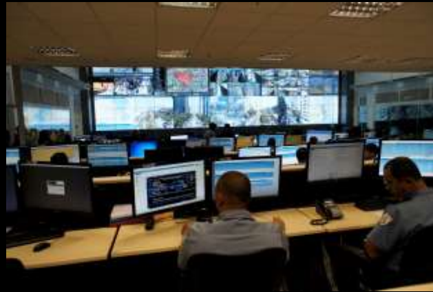
ICC Control Room Rio (military)
