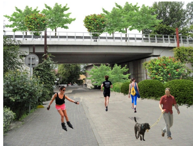
Fig.9. Street under the viaduct
