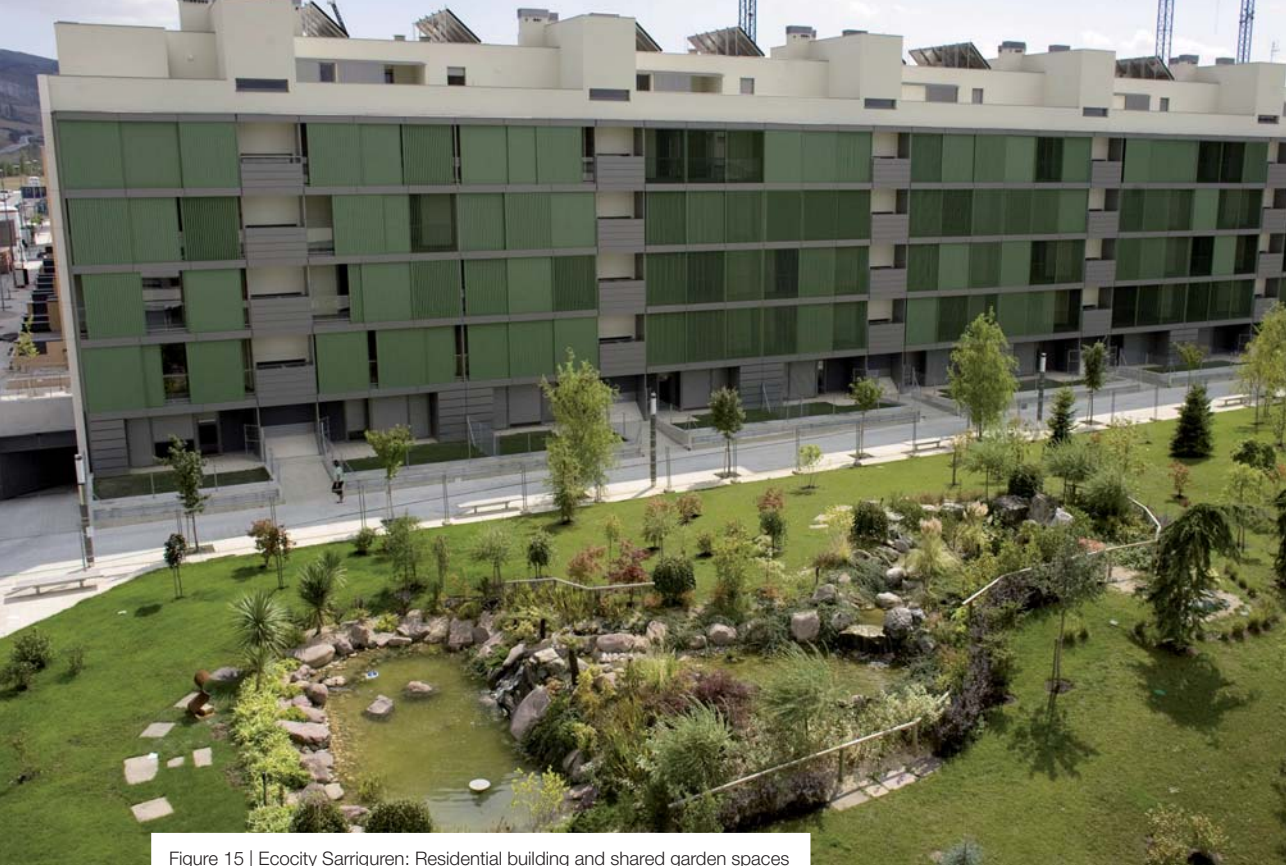
Figure 16 | Ecocity Sarriguren: Residential building with louvered façade for solar protection
