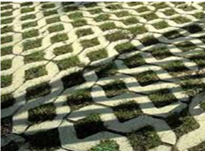
Installation of paving with suitable water permeability features. Top layer infiltration rate > 1X10-4m/s.
