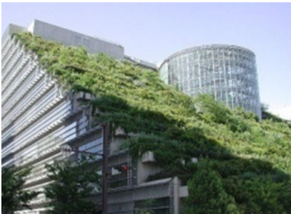
Planting on rooftop of building or structures. Green roof design consists of: water-proof layer, protective layer, drainage layer, purification layer and planting layer.
