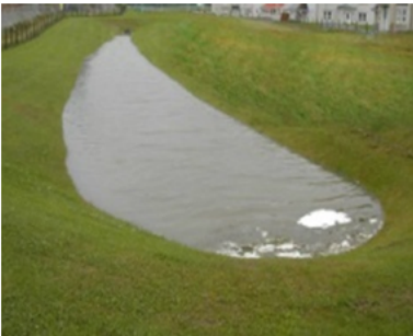
Designed for temporary or permanent detention of water to manage water quality. Depth of detention basin should be H=10cm.
