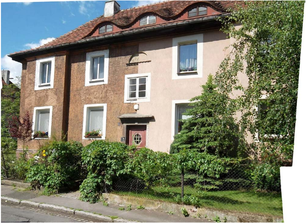
Image 2.1.3 Lost of original details when insulation is attached to external walls (Photo R Schuett)
