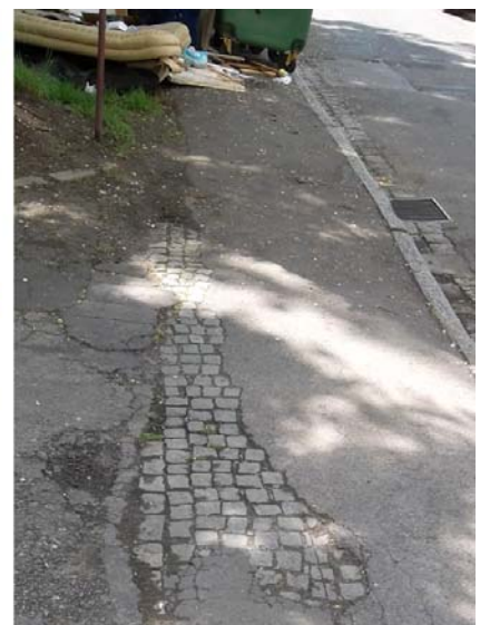
Image 2.1.7 Most of the original pavement (visible in some areas) has been covered with asphalt (Photo R Schuett)
