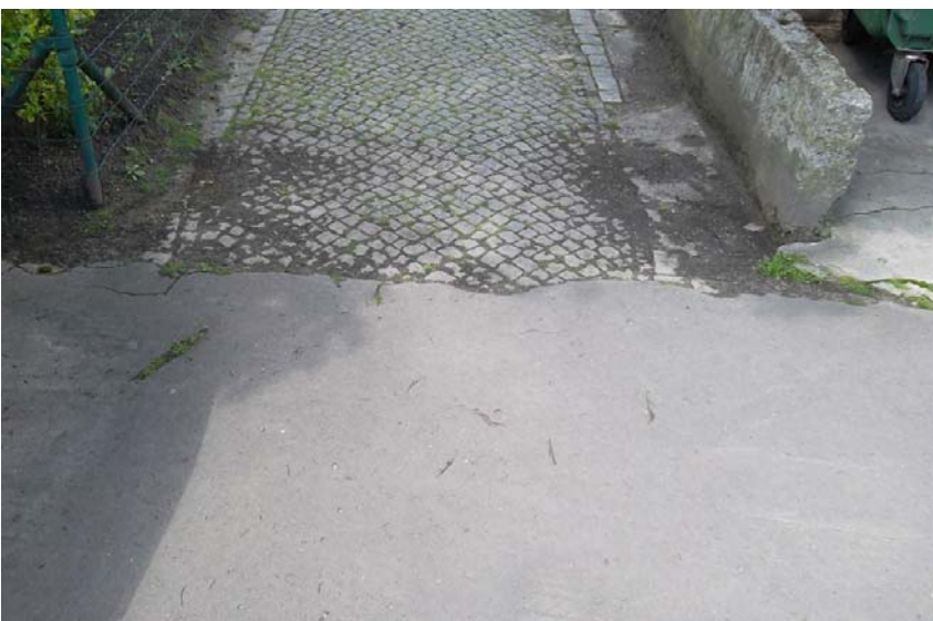
Image 2.1.7 Most of the original pavement (visible in some areas) has been covered with asphalt (Photo R Schuett)
