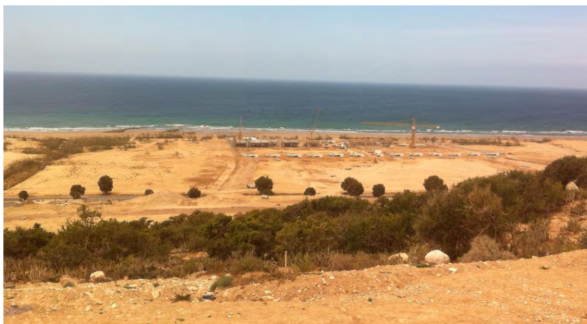
Figure 9: beginning of construction works (phase 4)
