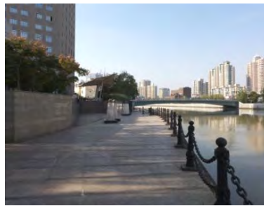
Figure 7: The stepped revetment
