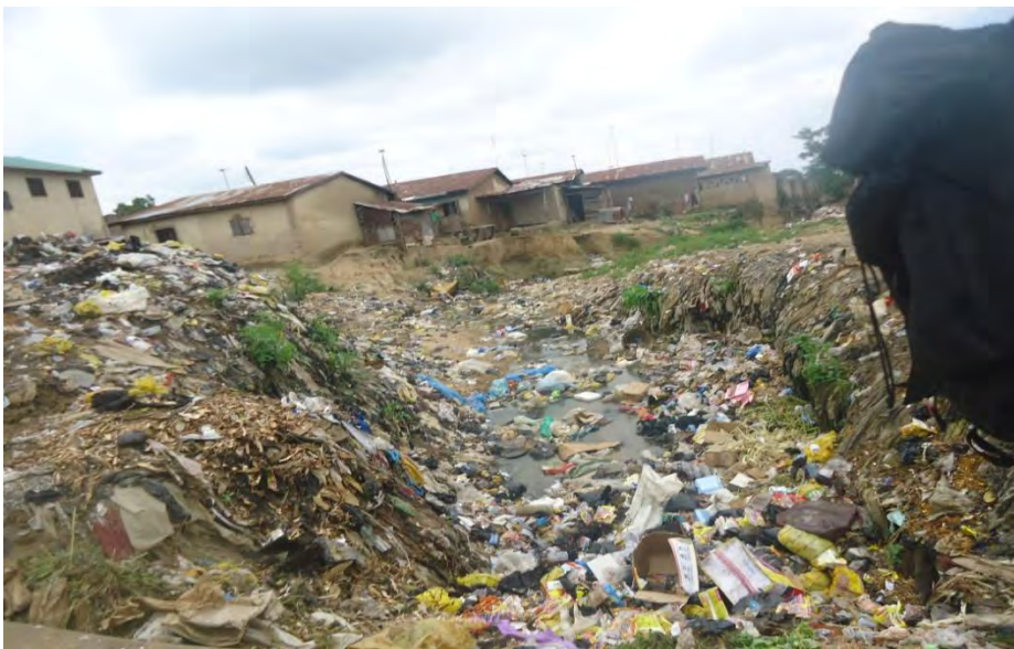
Plate 4.3: Buildings along waterways.
