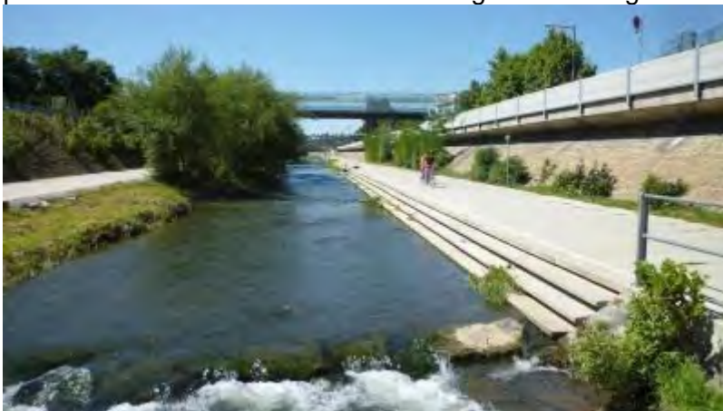
Fig.7 bicycle path next to renaturated section of the Wien River in the outskirts
