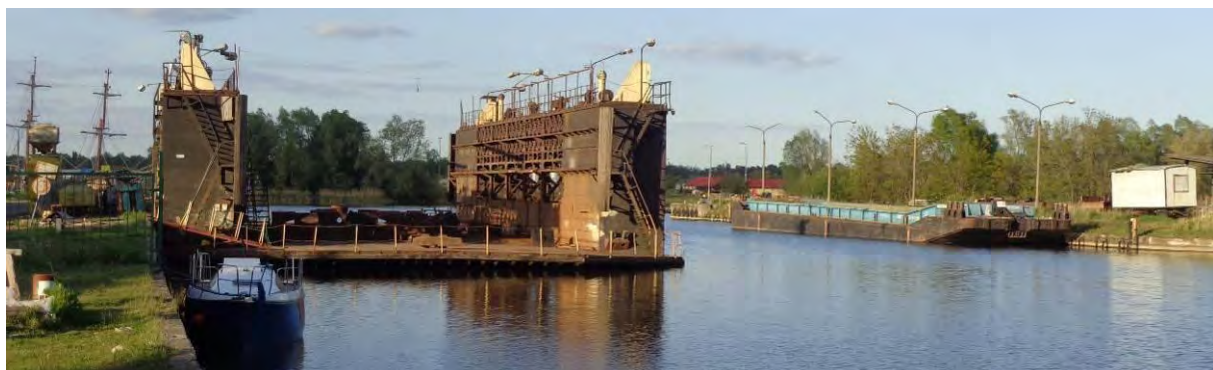
Figure 6: View of a floating dock built in 1880 (photo made by author 2014)
