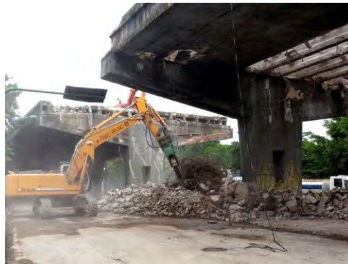
Figure 5: Demolition of the elevated expressway ( Perimetral )
