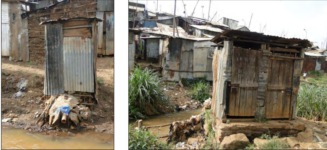
Plate 1: Toilet facilities located next to Mathare River
