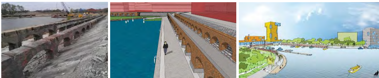
Image 13, 14 and 15: The construction of the quay wall in Hout dock, and two futuristic views, archive city of Ghent and sogent.
