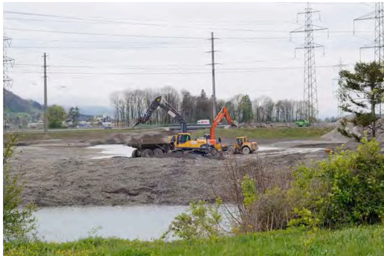
Figure 9: Improvements in progress. (© Author 2012)
