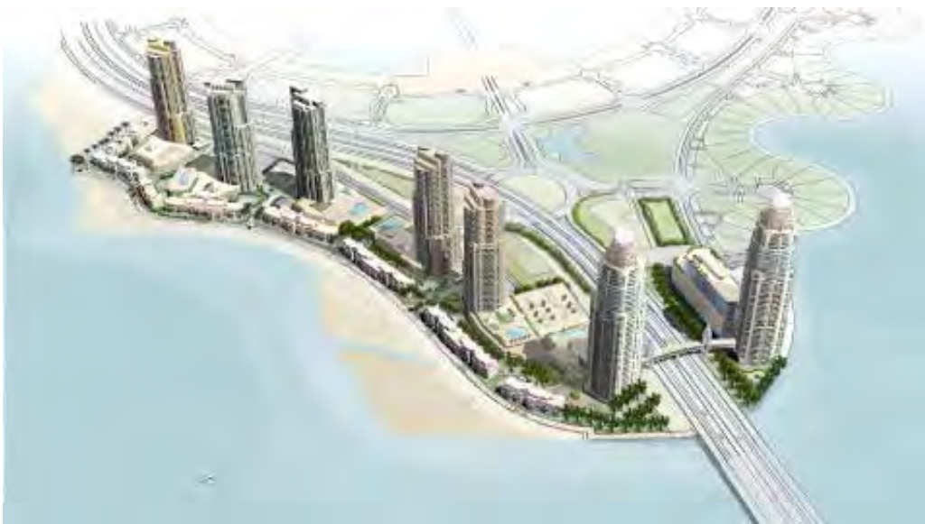
Figure 8. The Pearl: main gate development (source: The Pearl Advertising material).
