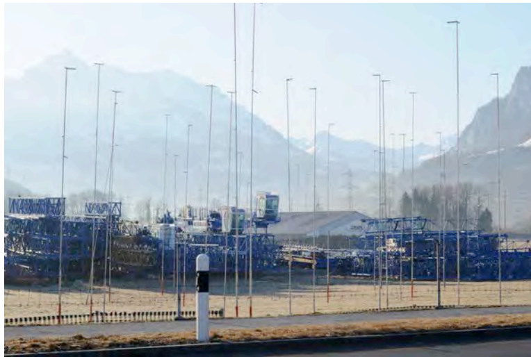
Figure 5: Development pressure in the Linth Plain, marked by construction profile boards that are required in order to obtain a building permit. (© Author 2012)
