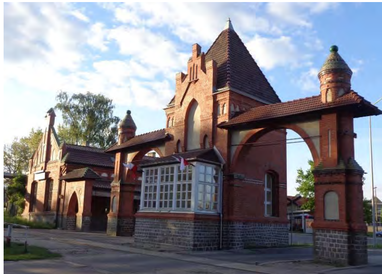
Figure 5: Main Gate to Free Port in Łasztownia (photo made by author 2014)
