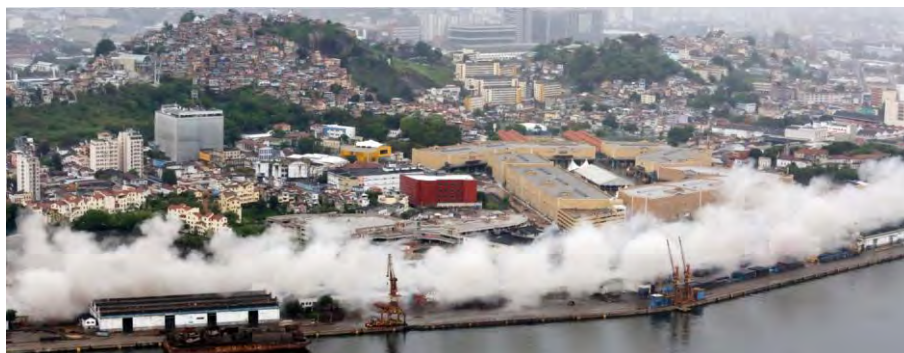
Figure 7: Demolition of the elevated expressway ( Perimetral )
