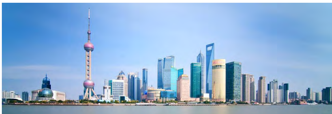
Figure 3: The Pudong skyline in east side of Huangpu River, Shanghai
