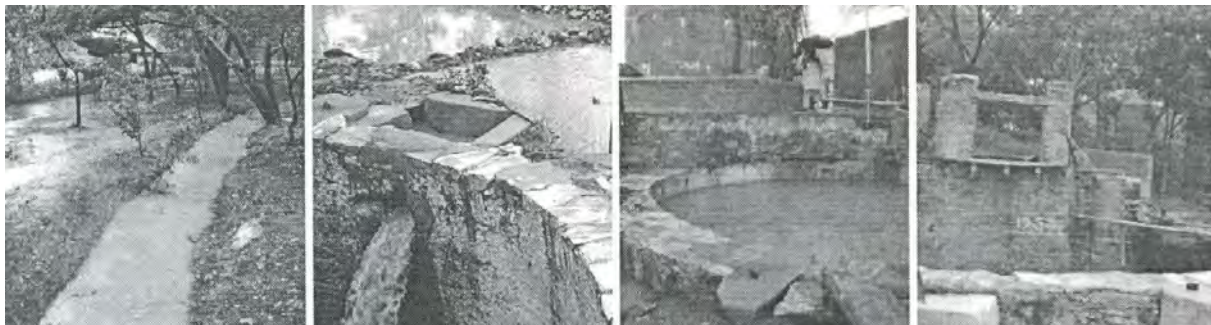
Figure 4: Trapping of Runoff: Figures above shows Channels and gullies are created to direct excess rain water into open wells and the water collects in the well. This water then percolates into the ground and within a week 3,00,000 litres of water percolates 100 ft. below ground level to recharge the ground water bodies.
