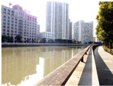
Figure 6: The vertical revetment
