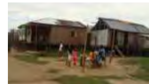
Fig.22 Houses on old riverbed, La Hoyada area,
