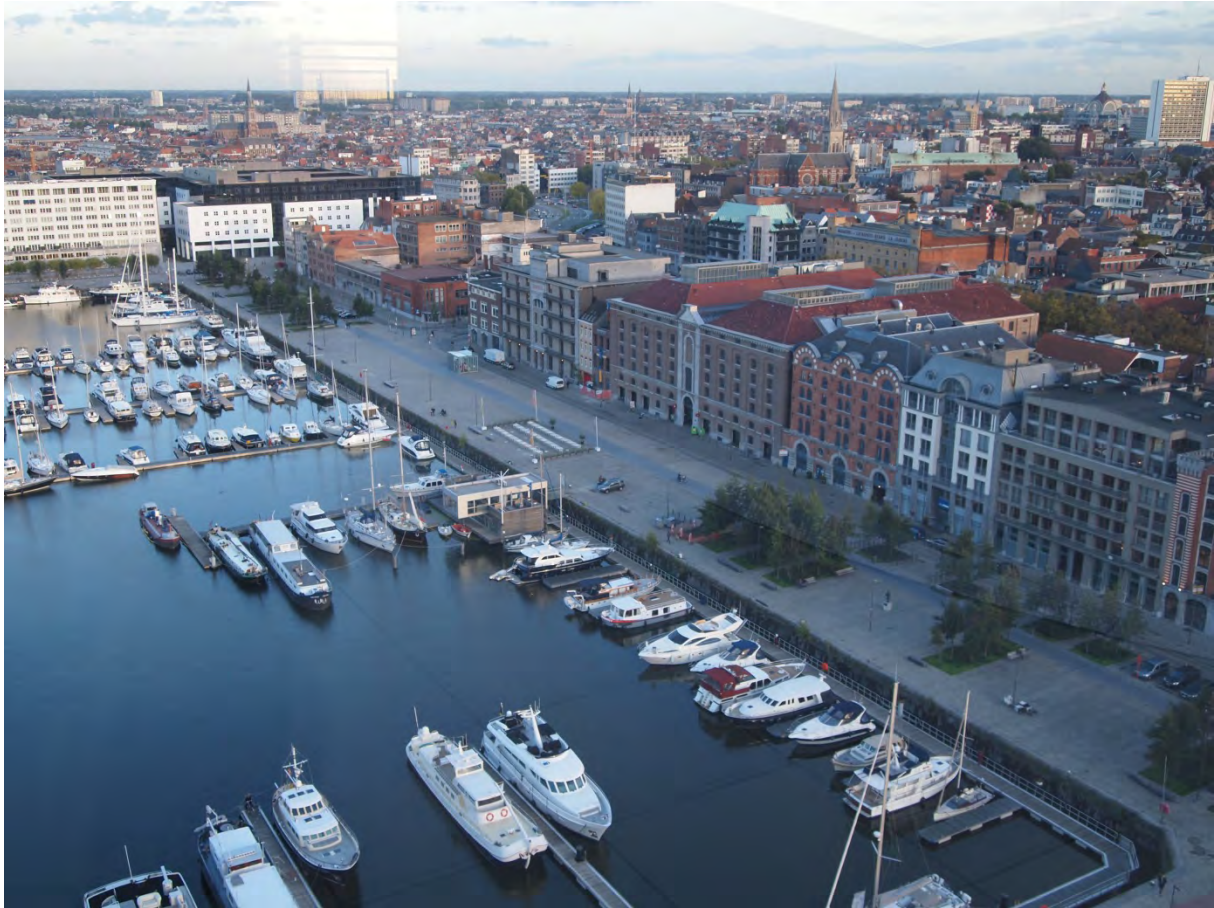
Redevelopment of public space along Bonaparte dock and Willem dock (the city's oldest two docks)
