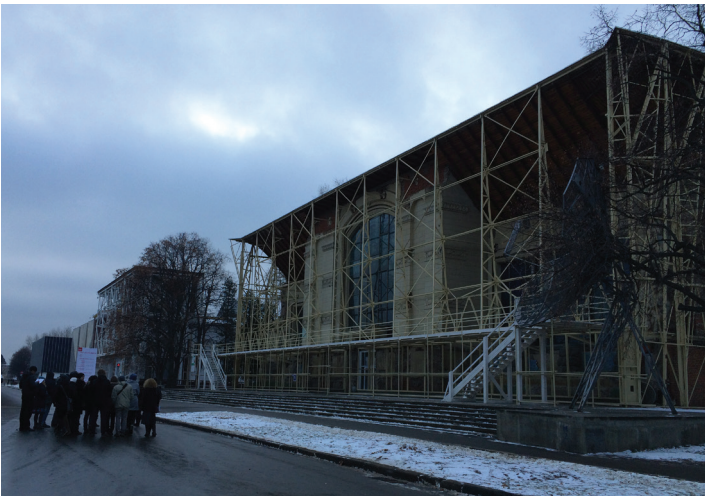
Some of the pavilions were renovated with modernistic covers with the old façades still present.
