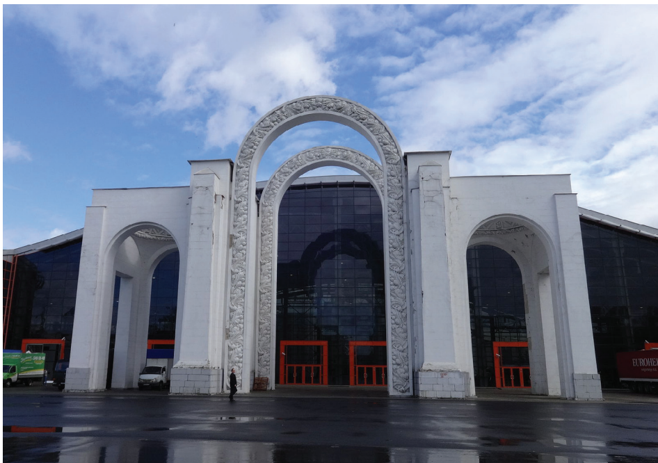
The former entrance gates of the exhibition of 1939
