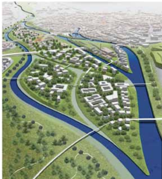
The Dutch office Kuipercompagnons advised to reopen and reuse former riverbeds of the river Warta for water catchment. The illustrations show low and high water level.
