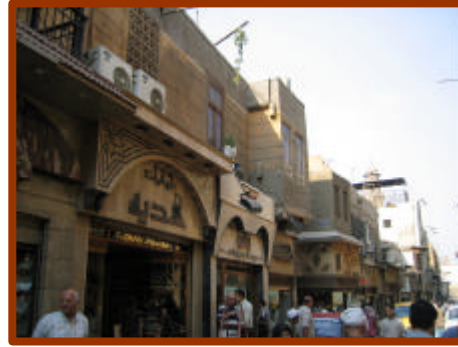
Figure 3a: Existing Façade Conditions
