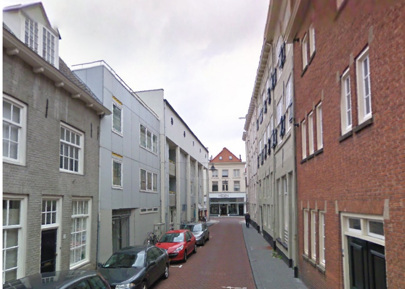
's-Hertogenbosch, small-scale filling, adapted to the surrounding buildings, which leaves the allotment intact
