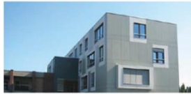
renewed office of the Port Authority: one of the first passive office buildings in Flanders (8)
