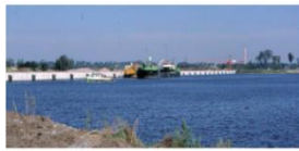
building a new dock with deep-water quays (2)
