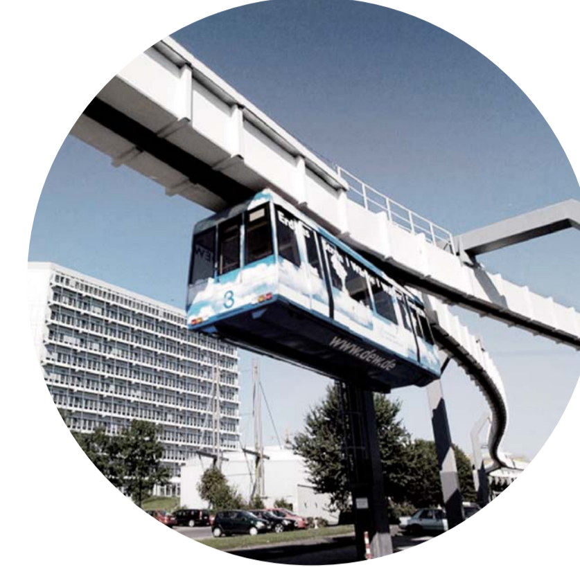
Renovating Infrastructure: Sustainable Urban Systems
