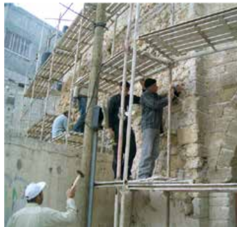
The Restoration of some residential buildings, Gaza (Done by IWAN, 2007)
