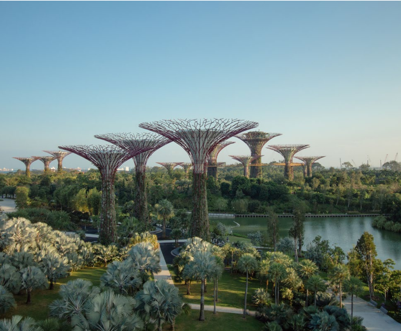
Figure 11: Singapore's Super Trees show the development of new and interesting hybrid forms of human-designed nature. These metal structures incorporate thousands of living plants and perform many of the functions as natural trees. Image credit: Singapore Nparks
