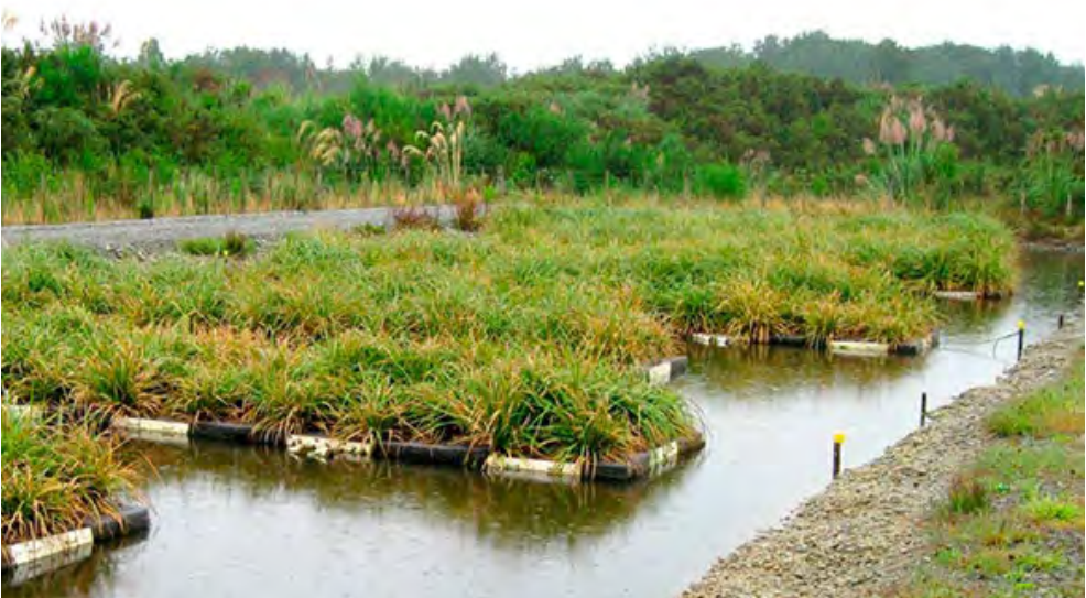
Fig. 4.1.13. Floating islands used as a measure to improve water quality Source: http://www.floatingislandinternational.com
