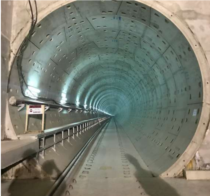
Figure 3: MRT Tunnels (Photo credits: Simarmata, 2018)
