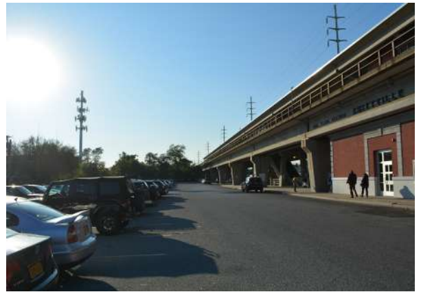
Figure 8: A commuter rail station in Long Island today
