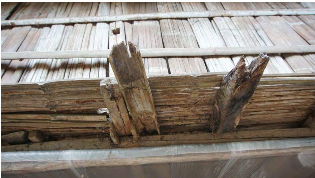
Figure 8 Yunnan Xishuangbanna Dailou uses wood and bamboo raft as building materials (Photo by Chen Lin)
