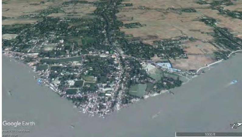
Figure 2 Google view of Chalna town showing Chalna canal in the middle
