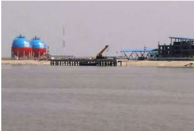
Figure 4 Natural Liquid Gas plant at the south of Chalna
