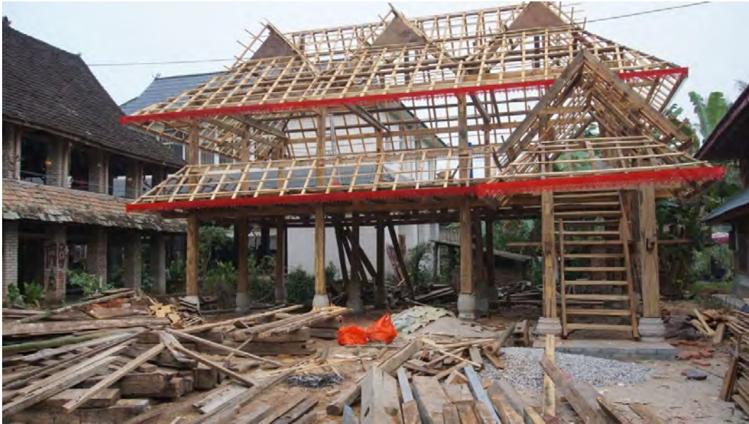
Figure 16 Dai people bamboo building construction skills(Photo by Chen Lin)
