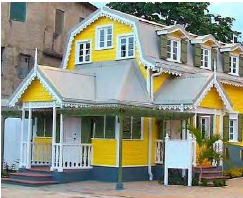
Figure 6a: Restored Derek Walcott house iv
