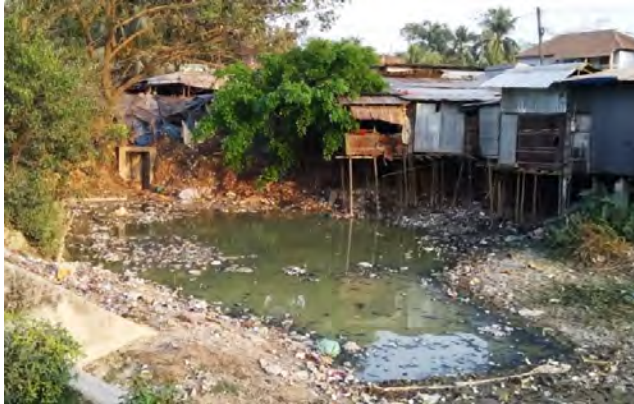
Figure 3 Dried up Chalna canal at inner side of the polder due to non functioning sluice gate
