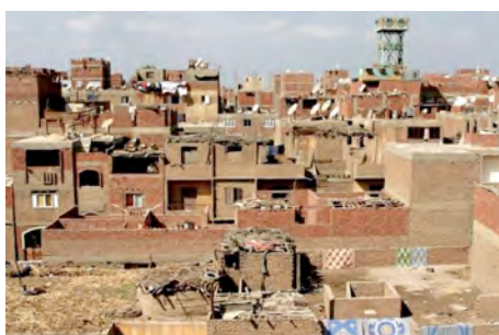
Figure 1: Illegal construction in existing residential neighborhoods 3
