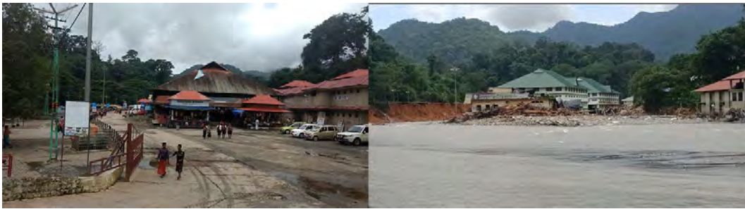
Figure 10. Before and after - Waiting area
