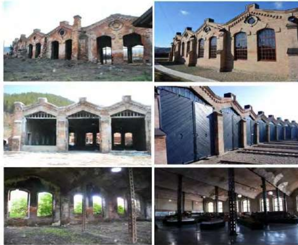
Figure 3 Comparison before and after repair of engine house
