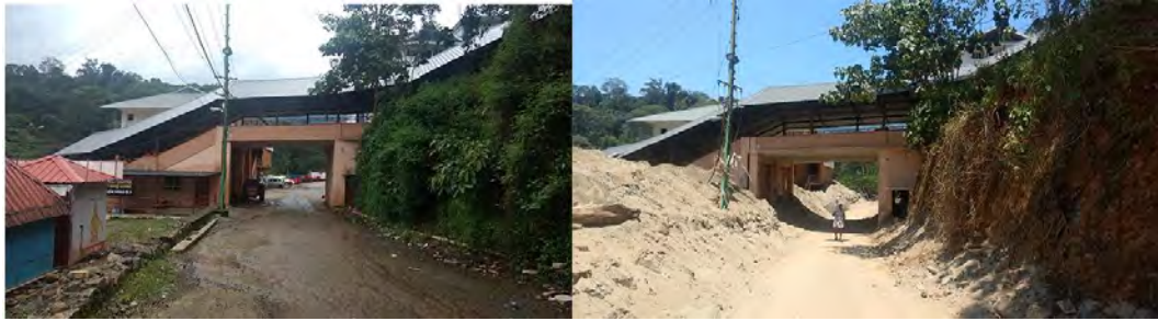
Figure 12. Before and after - Temple bridge
