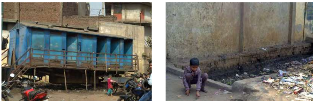
Figure 9: Ill maintained facility with sewage deposited flowing the facility in a space which is not distinct from recreational space for the children of the cluster
