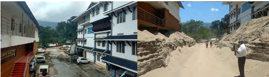
Figure 8. Before and after flood - Hospital
