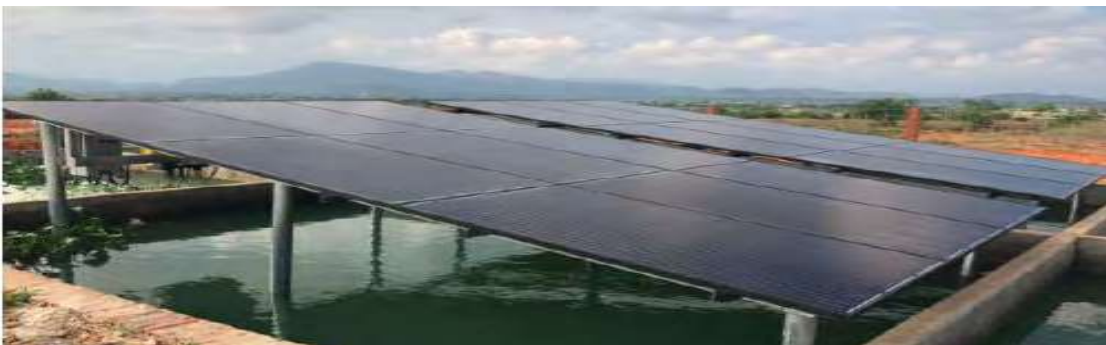
Picture 3 Solar energy used for aquaculture farm in Phu Lac.
