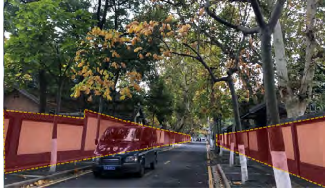
Figure 13 Closed street interface (Source: Drawn by project team)
