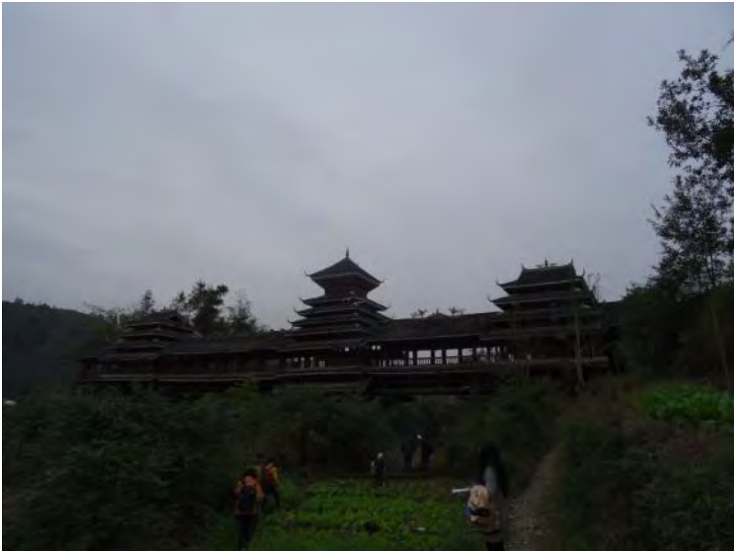
Figure 2 Guizhou Dong people's wind and rain bridge(Photo by Chen Lin)
