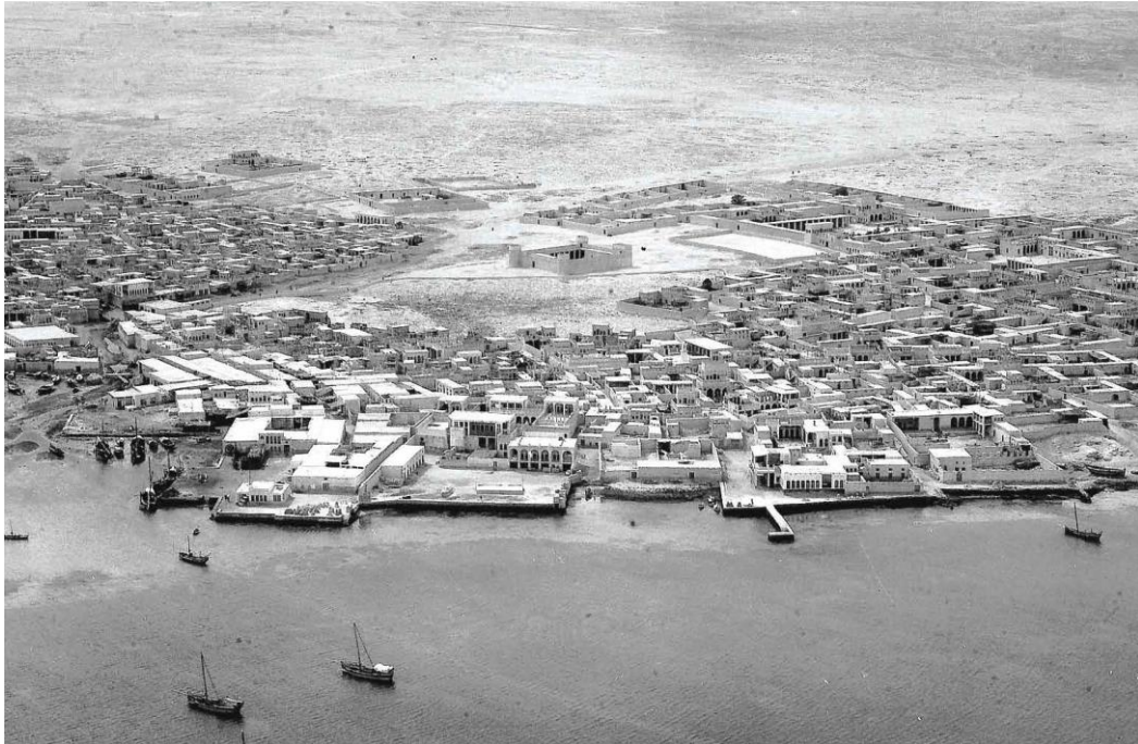
Figure 2: An aerial photo captured in mid-forties showing Doha's waterfront, AL Jessra Area, the cemetery and Al Khot Fort (Source: Ministry of Municipality -MME).
