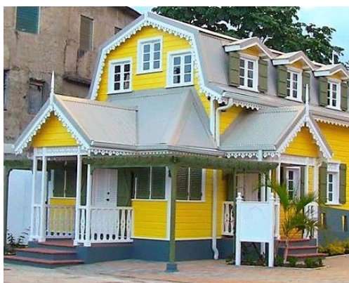
Figure 6a: Restored Derek Walcott house iv
