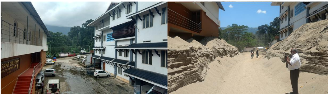
Figure 8. Before and after flood - Hospital
