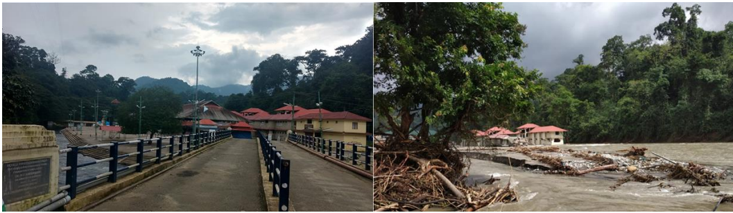
Figure 9. Before and after flood - Bridge
