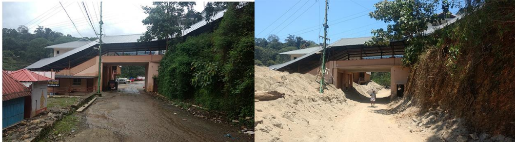
Figure 12. Before and after - Temple bridge
