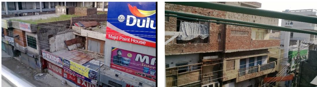
Figure 10. Exposed roofs and facades along the elevated route (Source:Author)
