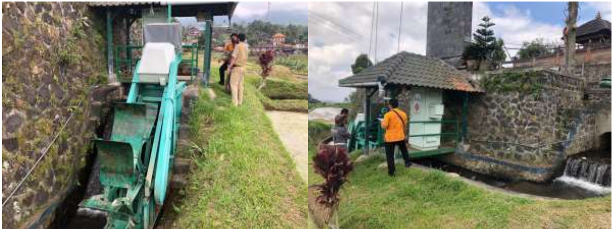
Figure 3. Piko hydro using Drainage & Irrigation system (Subak) in Jatiluwih. Source: field survey 2020.
