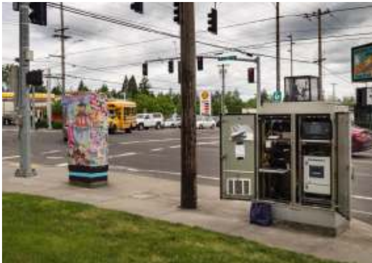
Figure 9: The City of Portland Curbside Lab for Emissions and Atmospheric Research cabinet on the right at the intersection of SE 122nd Ave and SE Division St. The traffic signal cabinet operating the signals and decorated with community art is on the left
