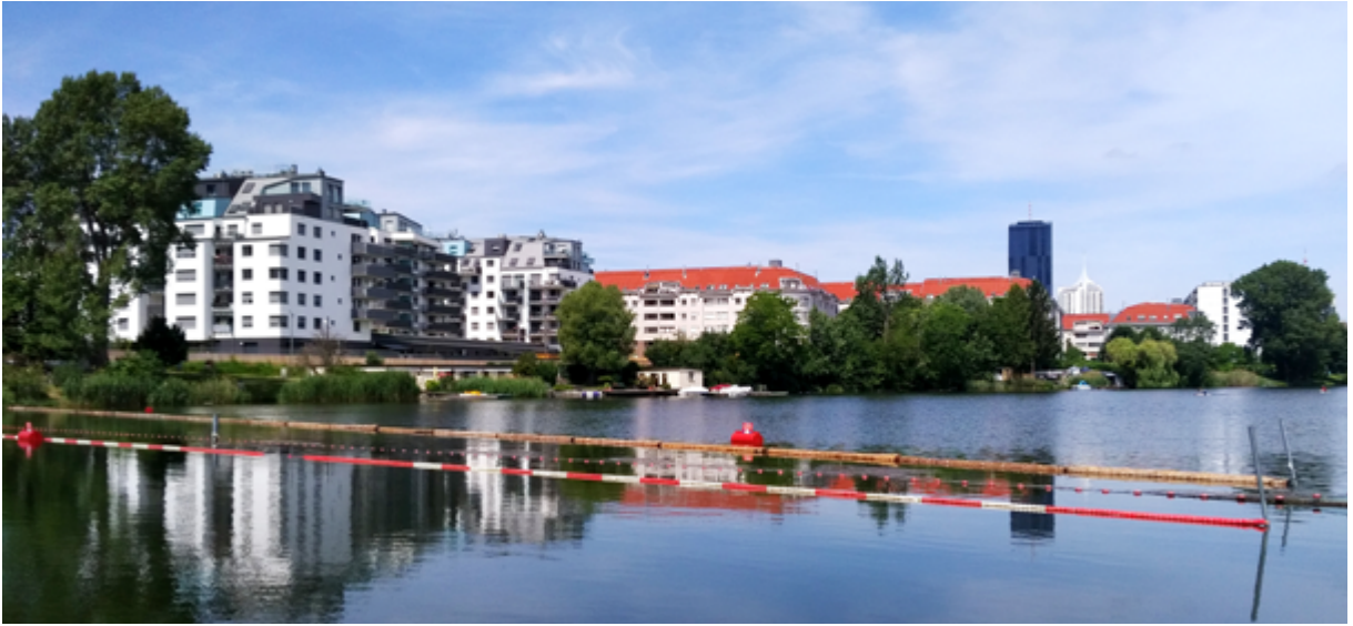
FIGURE 14: Attractive settlement areas, mixed with social housing, along the Old Danube
