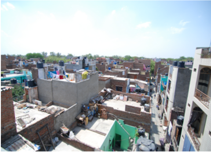
FIGURE 7: Mongolpuri - A Type D resettlement Colony in north Delhi. The majority of 7x3 meters units are already multi-story, built incrementally over the last decades
