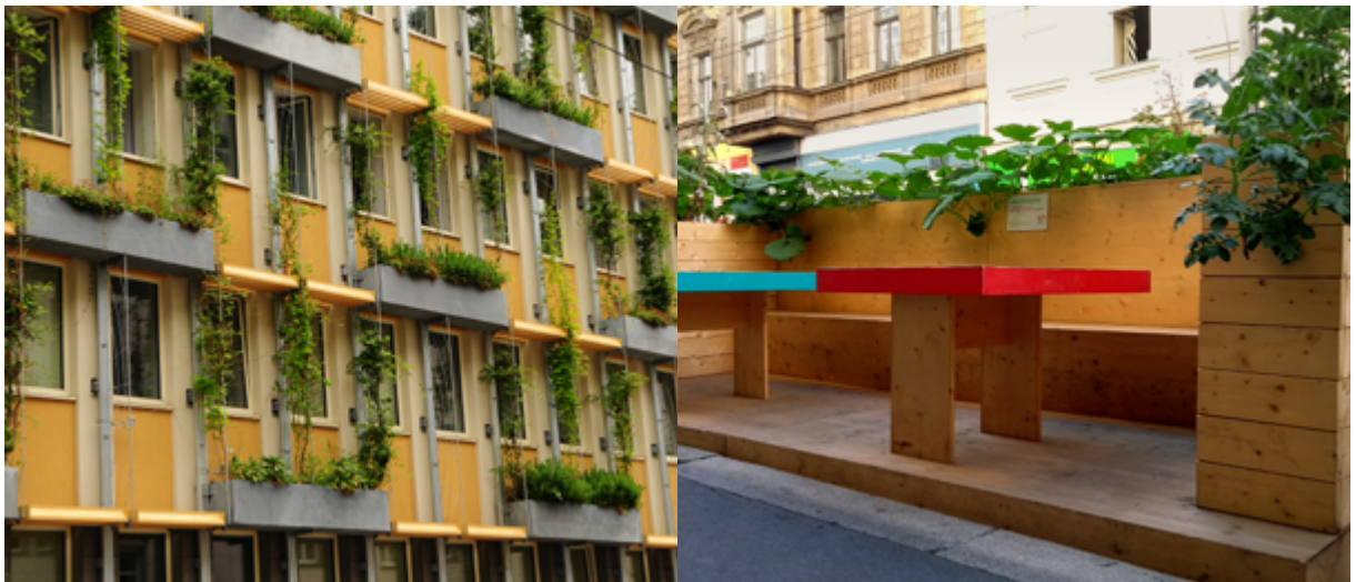
FIGURE 12: As space is scarce, Vienna begins to use vertical surfaces for greening. Façade greening of a public building (MA31)
