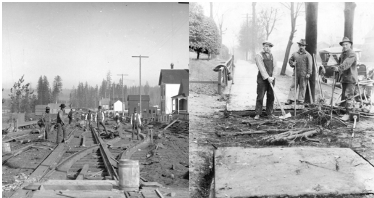
FIGURE 15 AND FIGURE 16: Vancouver's earliest roads were built by hand and street trees were planted into soils with relatively intact structure and less compaction. Trees planted into these early streets were able to grow their roots in soil under roads and sidewalks. Even today it is not uncommon to find the roots of mature trees under old sidewalks or roads when they are being reconstructed. SOURCE: City of Vancouver Archives
