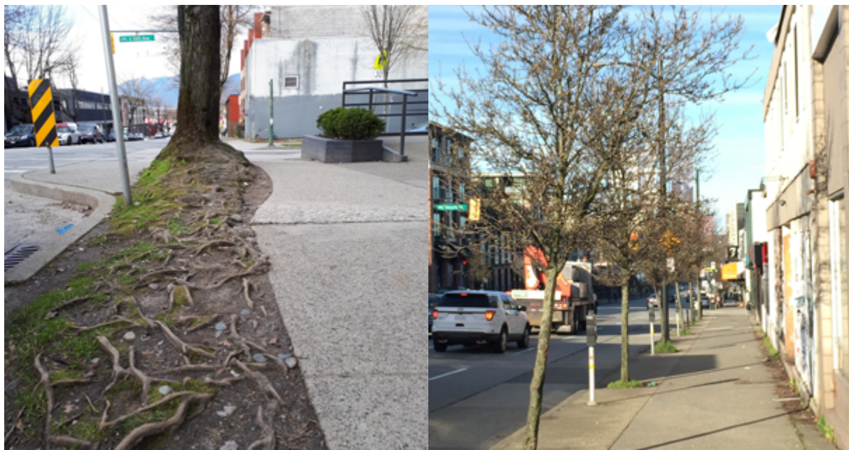
FIGURE 13 (SOURCE: Camille Lefrançois) & FIGURE 14 (SOURCE: Amelia Needoba): Street trees are often planted into degraded growing sites with compacted soil and low permeability. Where roots grow can be a sign of these conditions. For instance, compacted soils can restrict roots to the surface, or to find opportunities to grow under sidewalks and in utility trenches where roots can cause conflicts.
