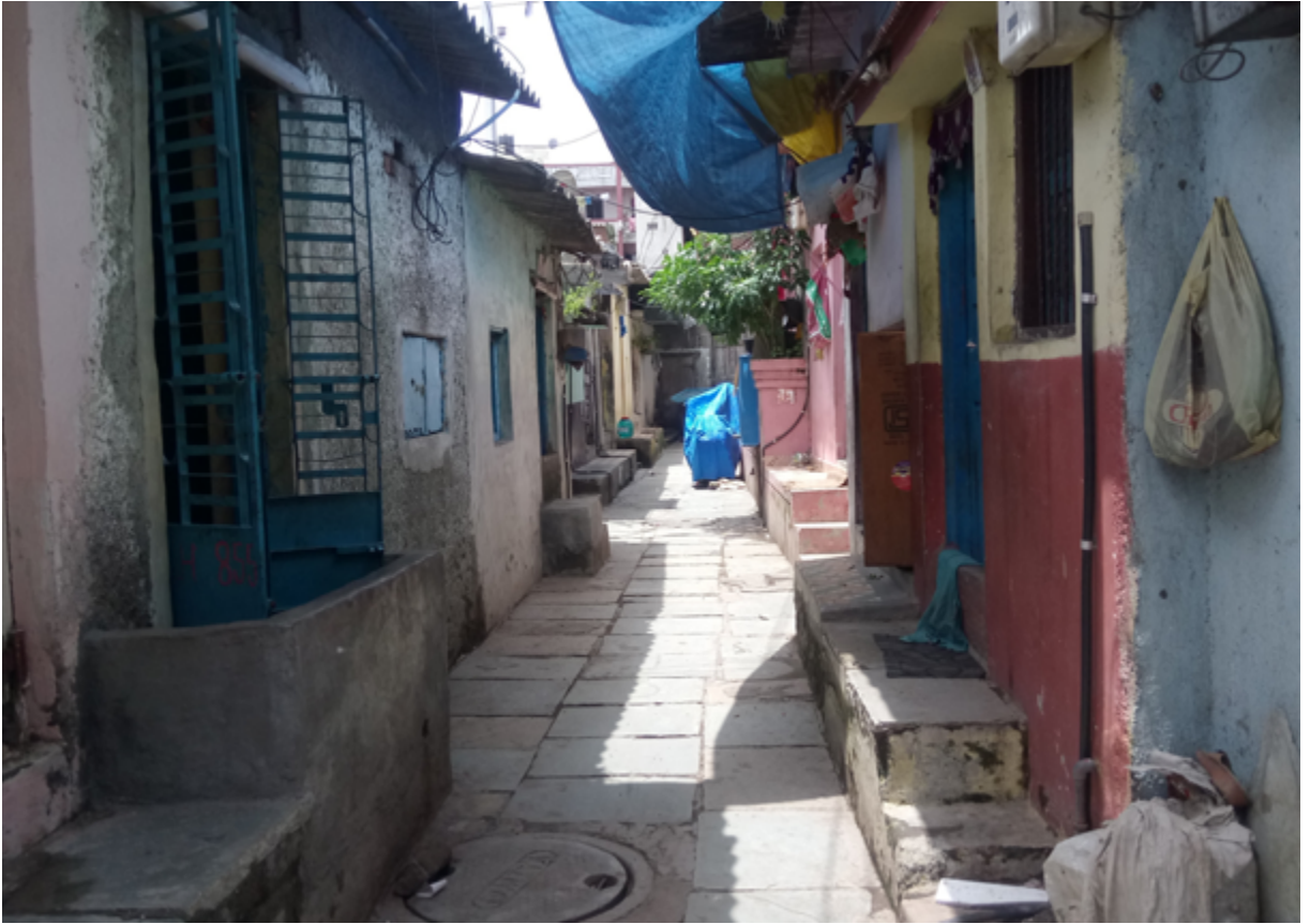
FIGURE 6: Street through the Morarji Vasahat slum community, showing elevated plinths and high doorway thresholds. Source: WRI India
