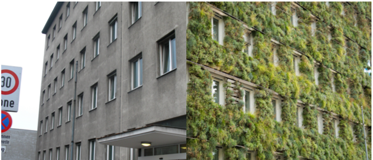
FIGURE 8: Green facades to shade and humify the rooms behind instead of air-conditioning on a MA 48 - Waste Management Department building. SOURCE: MA 22
