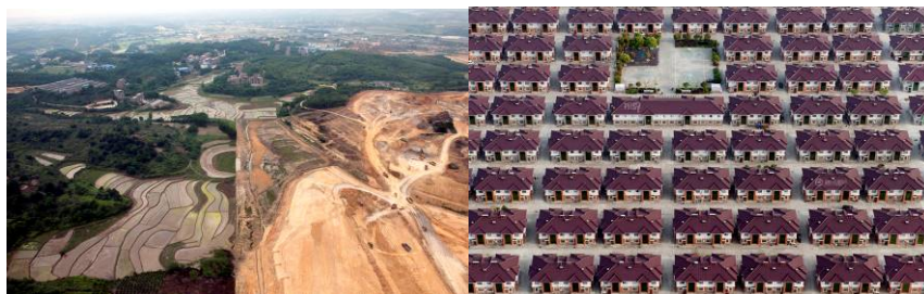
Figure 1: Damage to the rural landscape by simple and crude planning and design. Image Source: https://www.worldphoto.org/zh/node/1549
