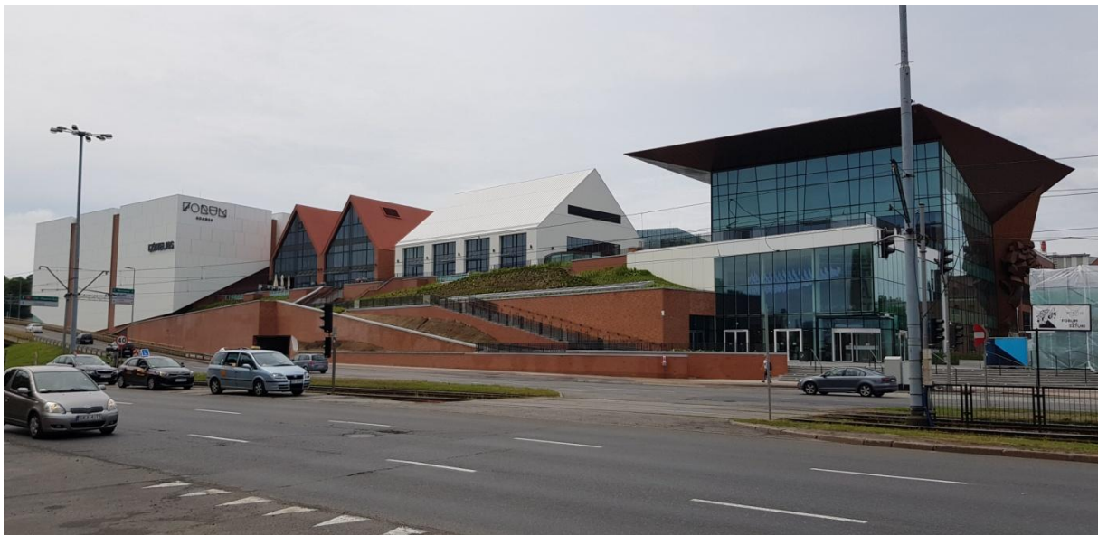
Fig. 3. General view of the Forum Gdansk complex (2018). Photo credit: M. Habier
