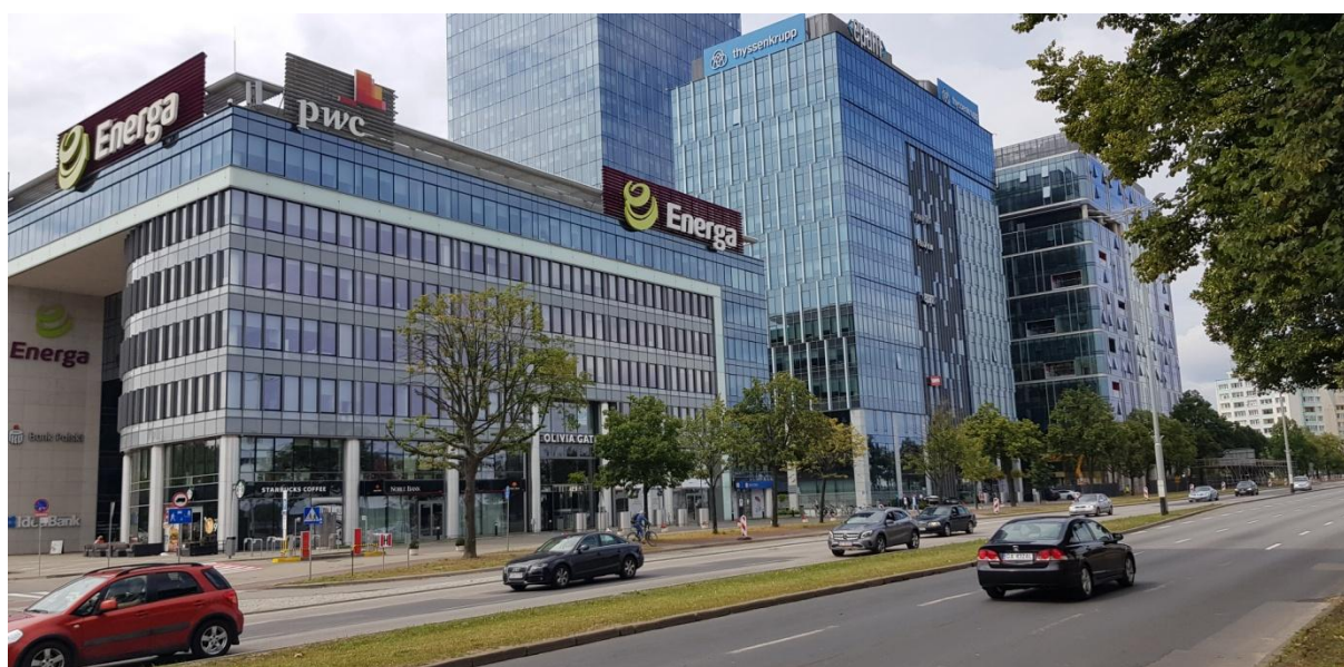
Fig. 6. General view of the Olivia Business Center complex (2018). Photo credit: M. Habier
