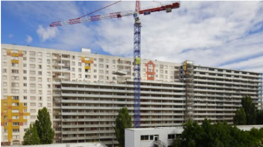
Figure 4. Transformation of 530 dwellings during construction work. Copyright: Philippe Rualt
