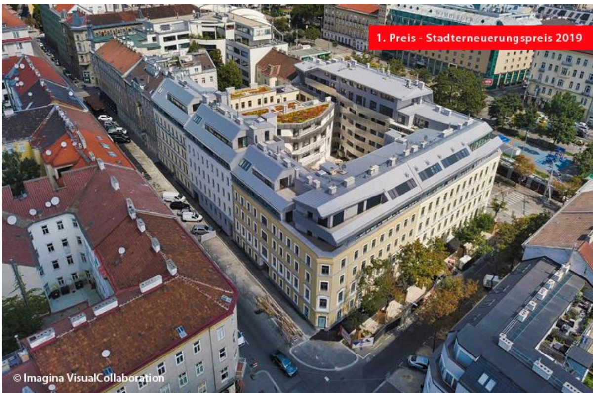
Figure 8. Refurbishment of a Gründerzeit housing block, Vienna Goldschlagstr. , with additions and greening, Source: PGood
