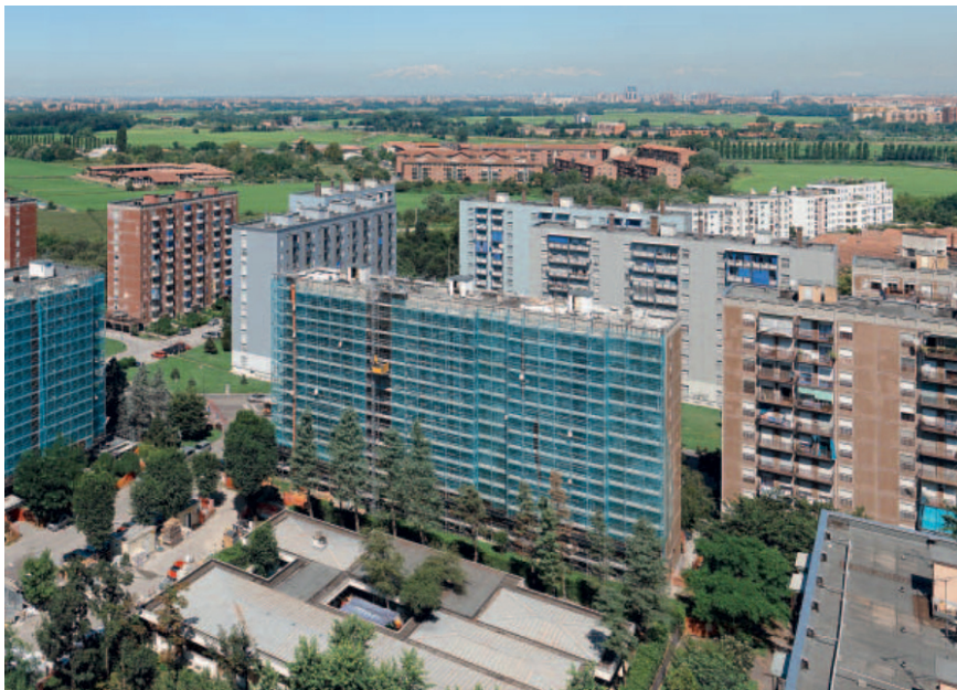
Figure 2. The buildings of Gratosoglio during the renovation. Source: Arketipo
