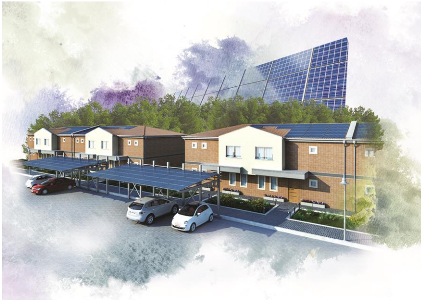
Figure 11. Rooftop Building Integrated Photovoltaic system plus Carport Canopy on the ground, source: Tepebaşı Municipality
