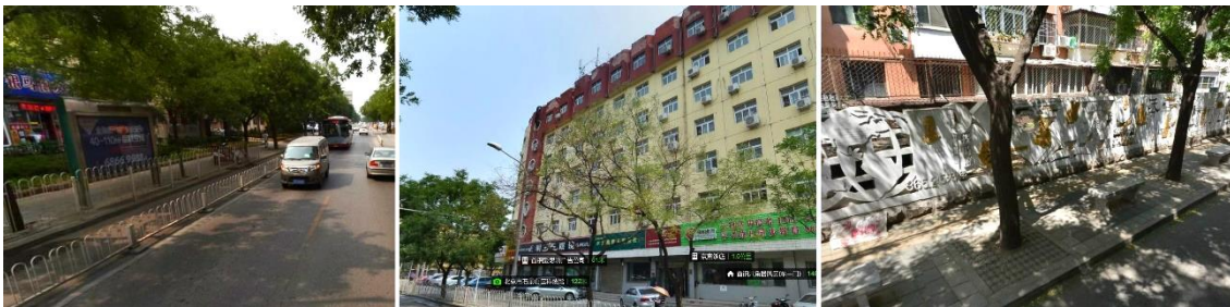
Figure 5 Separation fence, building façade and fence after the last round of remediation
