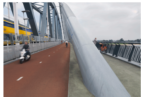
3.2.3.3 RijnWaalPad is a cycling highway that connects Arnhem with Nijmegen in the Netherlands. Different types of movement are separate from each other.
