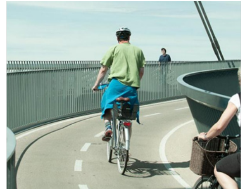
3.2.3.1 One of the cyclist-only bridges in Odense.
