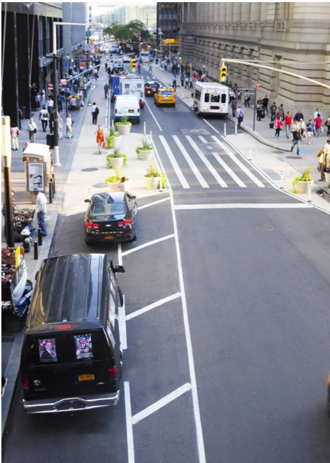
3.3.4.2 Curb extension of the sidewalk. It increases the overall visibility of pedestrians by aligning them with the parking lane and reducing the crossing distance for pedestrians (Bowling Green, KY, USA).
