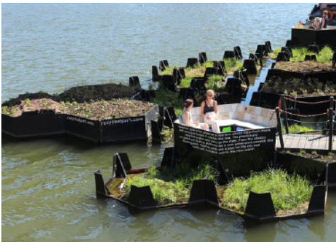
5.3.2. Floating recycled park in Rotterdam made out of hexagon elements from nearby collected and recycled plastic waste
