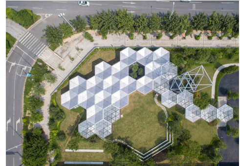
5.2.1. HEX-SYS - modular project, where a set of hexagons assembled together create a building and a pa-
