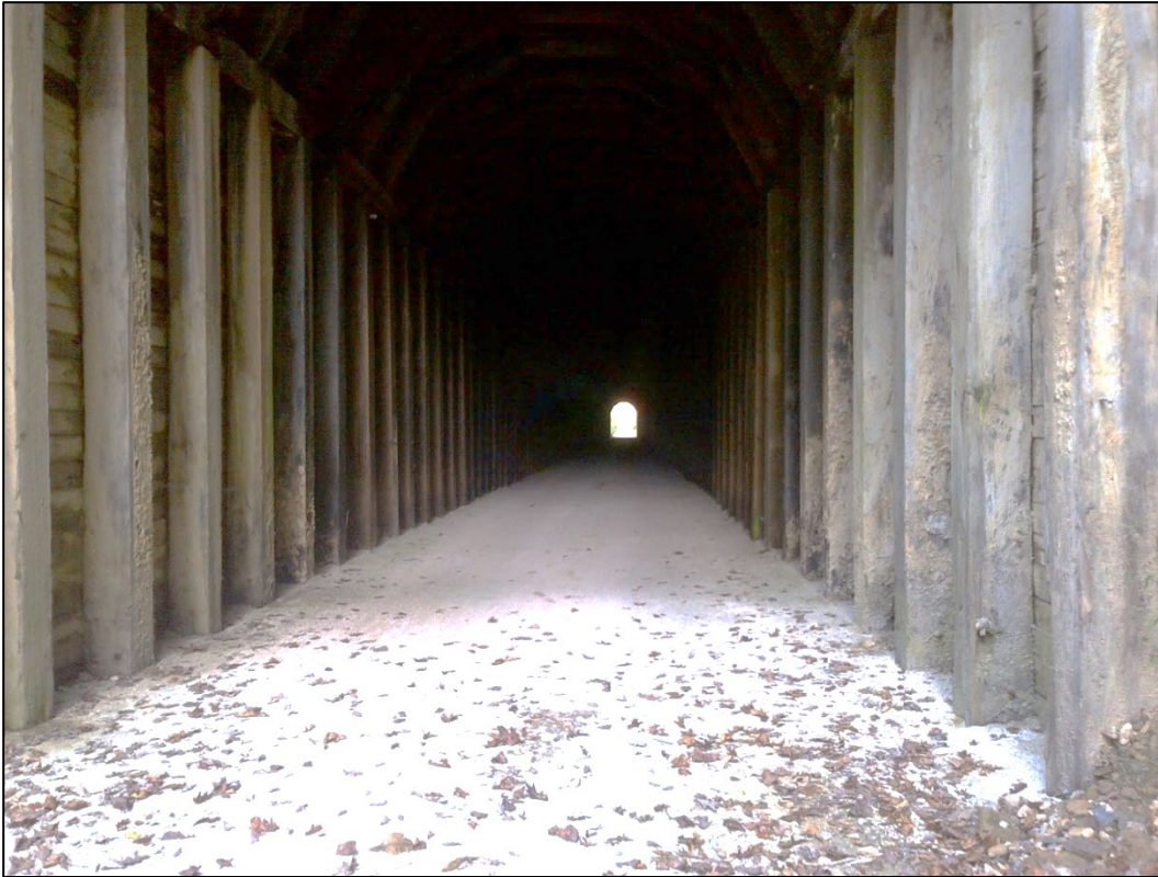
Pedestrian/Equestrian Tunnel – 600 ft. Long, Approx. 20 ft. High and 16 ft. Invert
