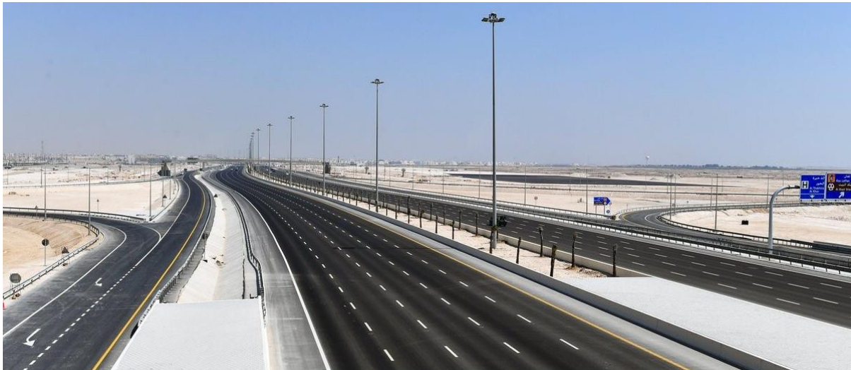
Figure 13. A Recently Built Expressway in Metropolitan Doha. Source: Ashghal. 113
