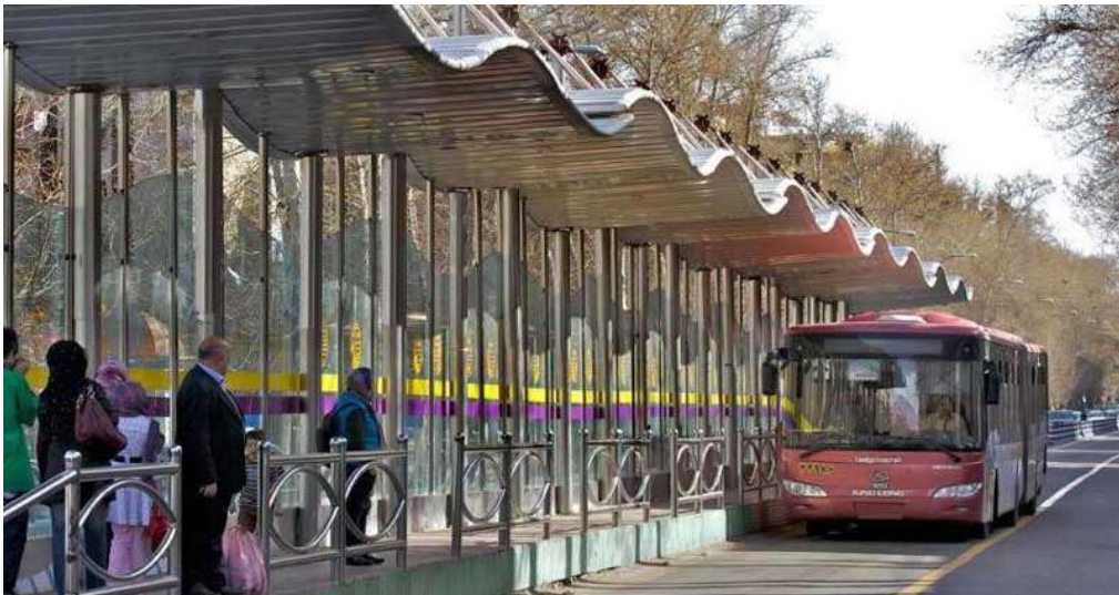
Figure 4 - The station of BRT of city of Tehran
