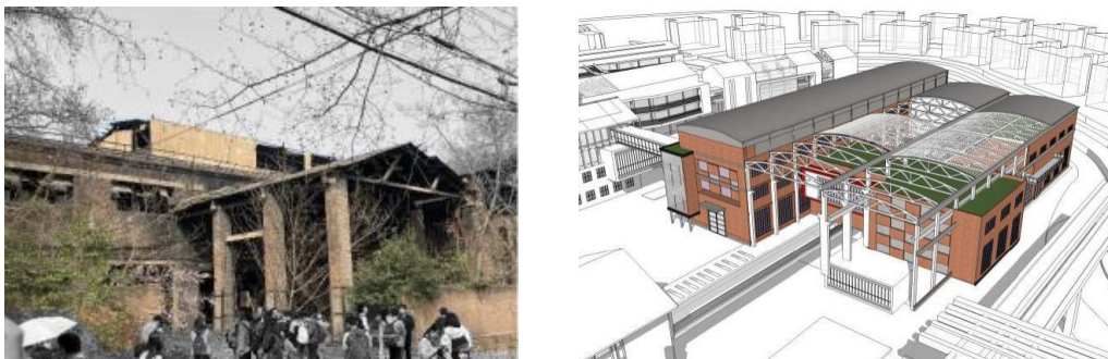
Figure 7. Expose old building structures. Source: By Author.
