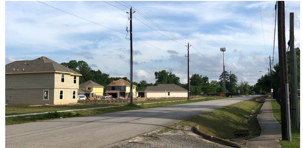
Figure 06 Open drain ditches in East Houston. Photo by author.
