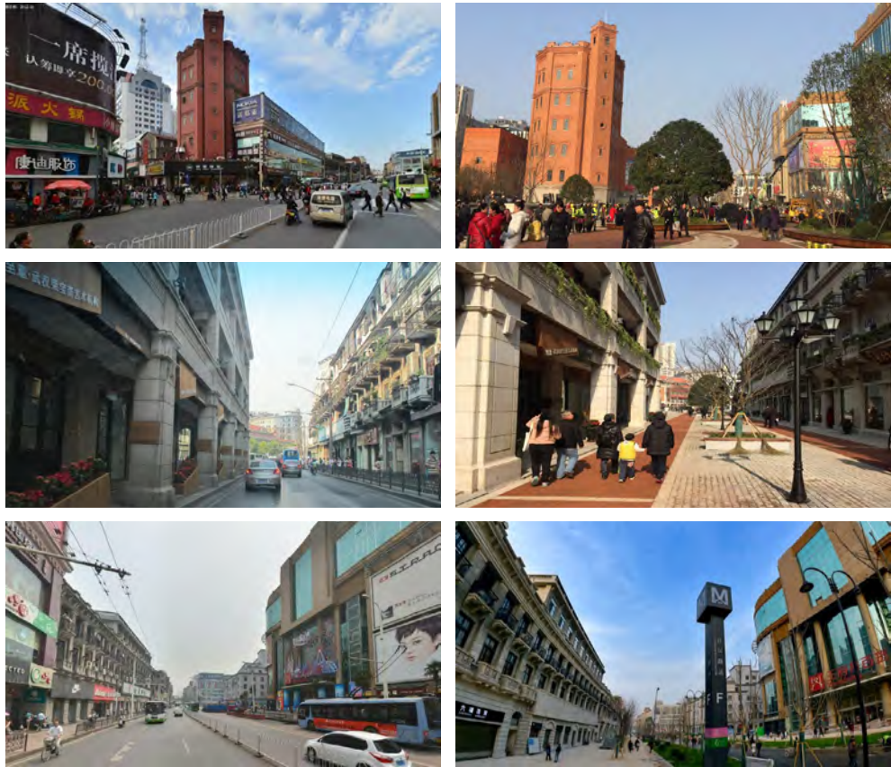
Figure 8: Before/After the Zhongshan Avenue Renewal Plan & Implementation. Source: WLSP
