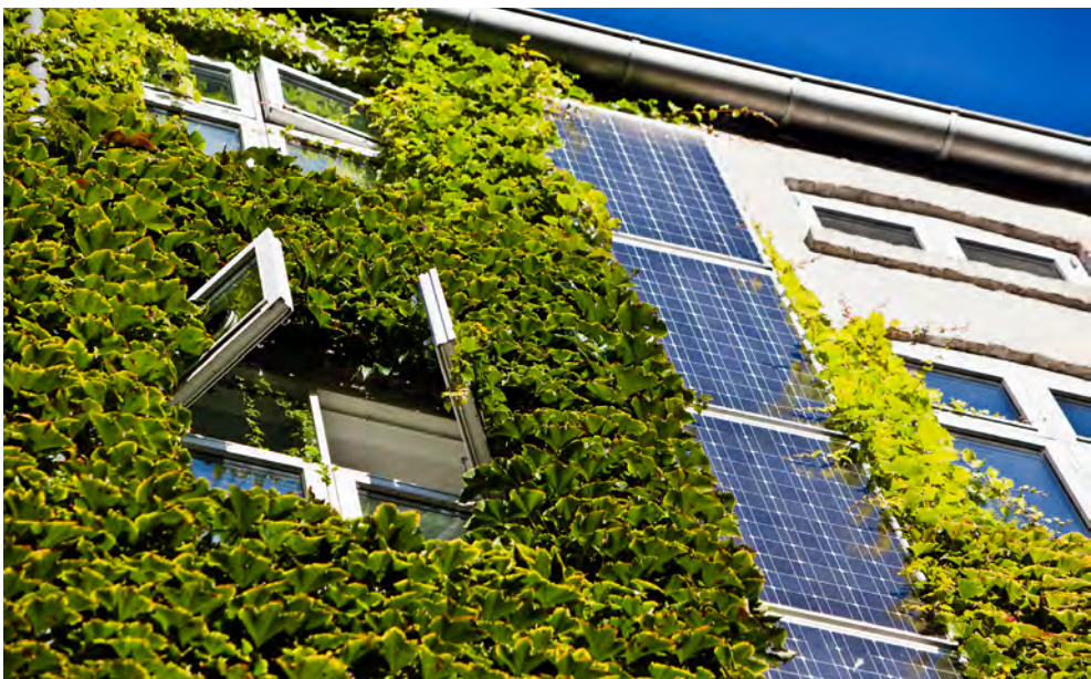
Figure 6: Energy efficient building in Copenhagen, Denmark. Source: The City of Copenhagen website www.kk.dk
