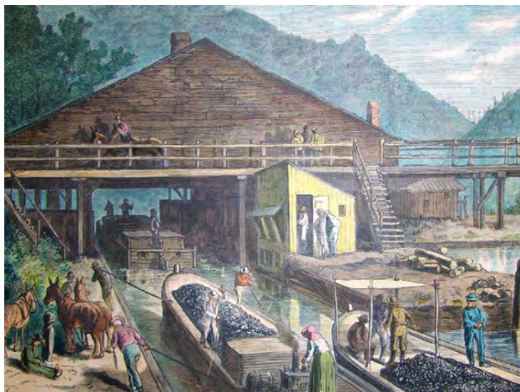
Figure 3: Illustration depicting Lehigh Canal Weigh Lock #2 near Mauch Chunk (present day Jim Thorpe, PA). Source: National Canal Museum Archives
