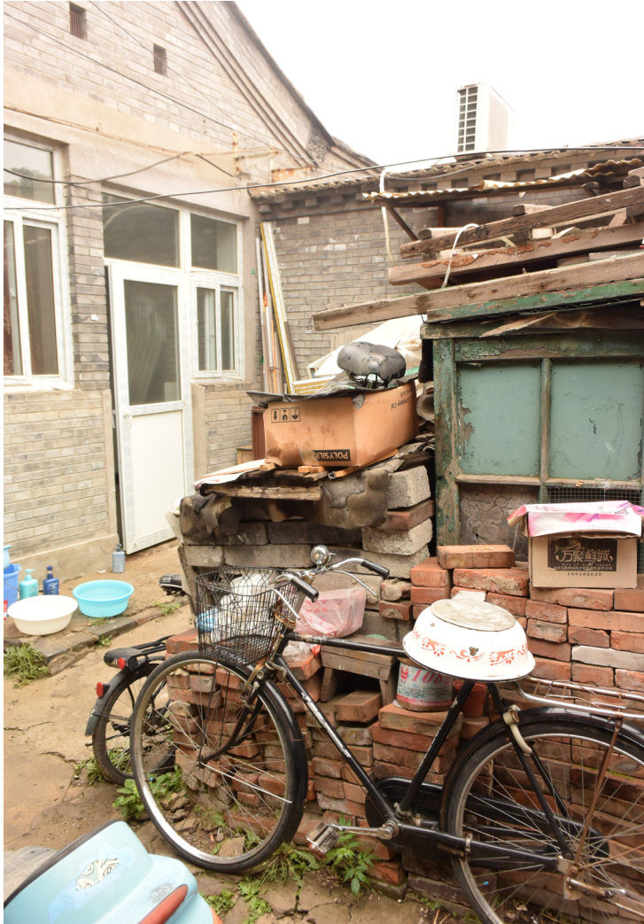
Figure 5: Current situations of “poorly-preserved courtyards”. Photo by Project Team
